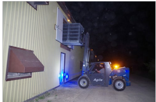
Figure 1. Forklift placing empty, 5-tier CM2A module into second floor.
